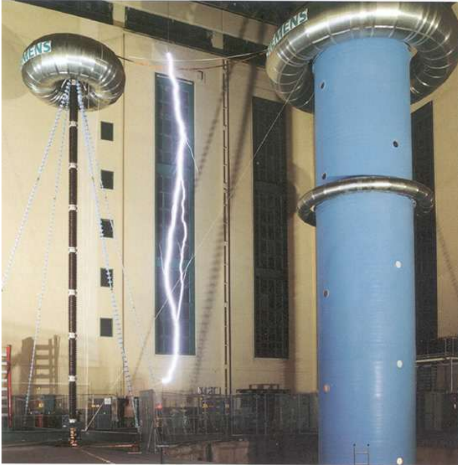
Fig 33.5 Damped capacitor voltage divider for 4.5-MV impulse voltage, outdoor
