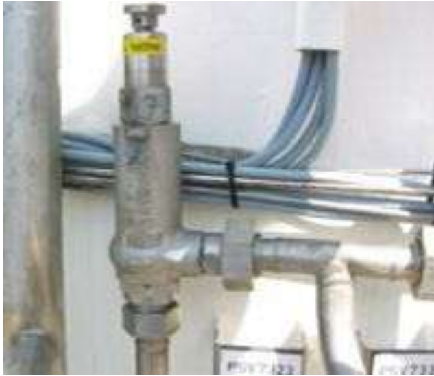
FIG – Oxygen Safety Valve
